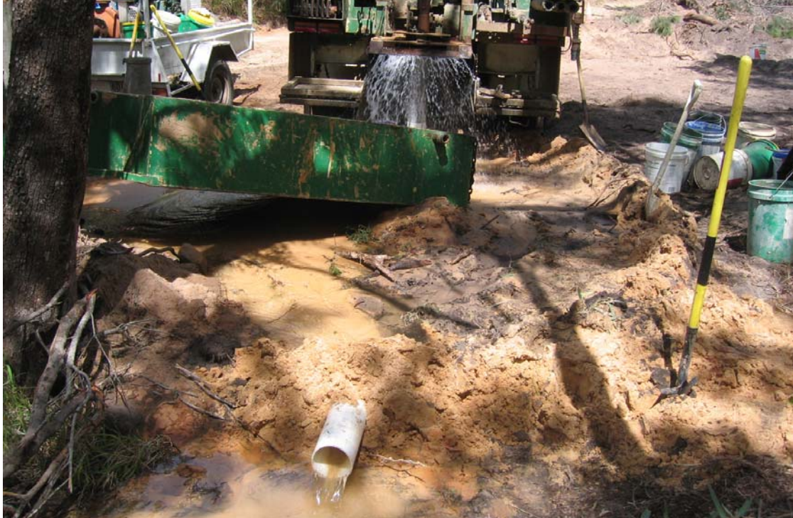
Photo 3: View of PB2 drilling site during the bore development and airlift flow test.
