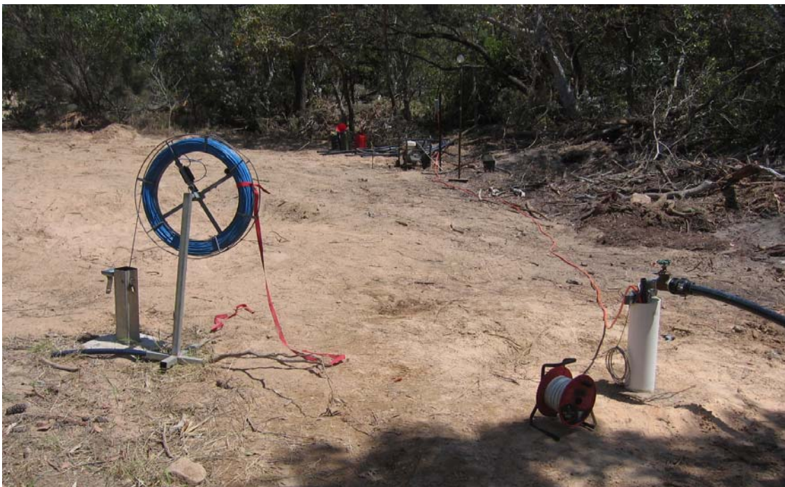
Photo 4: Pumping test carried out on PB1, Monitoring carried out in MB10 on the left and PB1 on the right.
