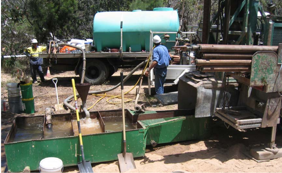
Photo 1: View of PB1 drilling site, mixing drilling mud and preparing to start drilling.
