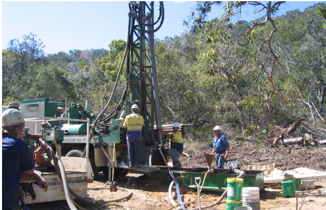
Photo 2: Installing the stainless steel screen into PB1.
